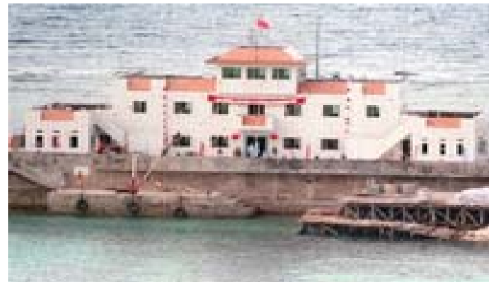
MISCHIEFS REEF HEADQUARTER AND LOGISTIC FACILITY (1)
