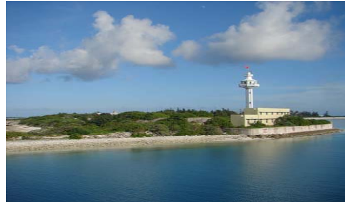
Duncan, Communication Tower
